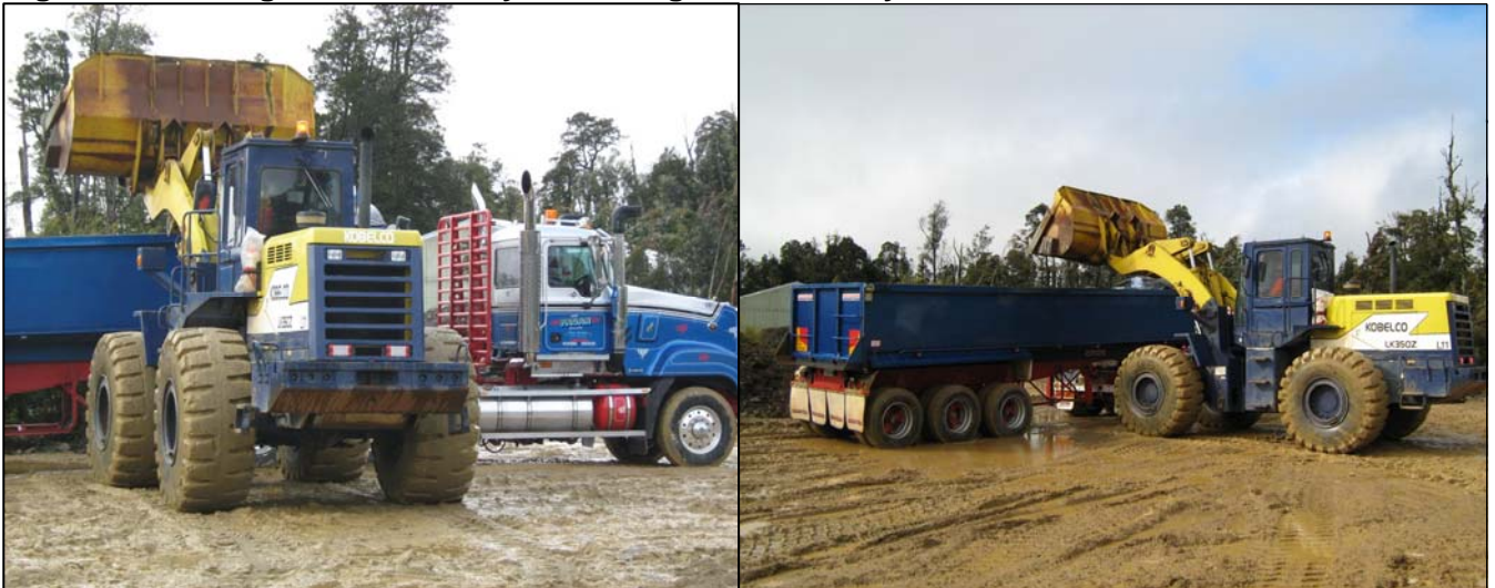
Figure 2: Loading of trucks ready for haulage to Rosebery
