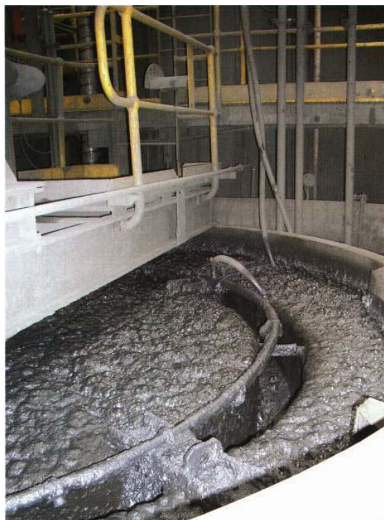
The Hellyer mill flotation circuit
